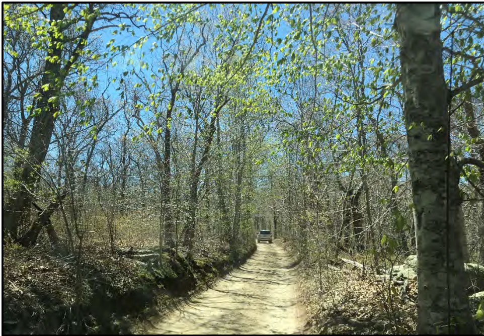
Figure A.1. Photograph showing the narrow unsurfaced road of a WUI community.
